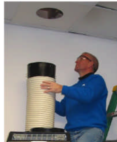
Extend duct and fit collar into opening.
