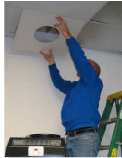
Place Ceiling Adapter into the ceiling grid.
