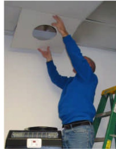
Place Ceiling Adapter into the ceiling grid.
